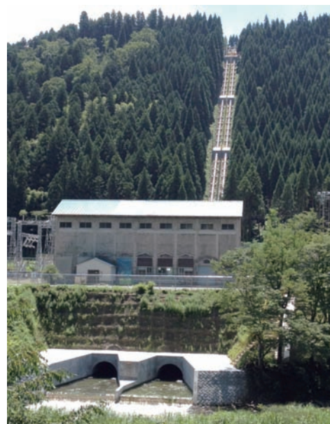
図5 小水力発電所の例 An example of small hydro power station
