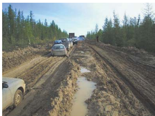
図2 劣悪環境地域の道路状況 Poor road conditions in environment area
