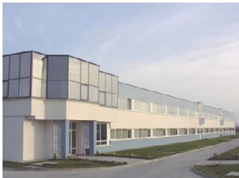
SNR Romania plant
