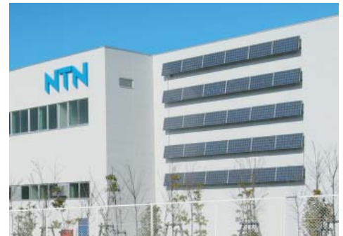
Photovoltaic generation at NTN Mie Corp. Plant No. 2
