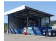
New waste storage center
