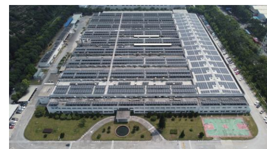
Power supply by solar panels (China: Guangzhou NTN)
