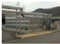
Thermal storage tank for hydrate-slurry air conditioning system (Okayama Works)
