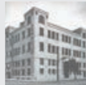
Old head office building
