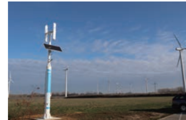
NTN Green Power Station (front) installed in NTN-AT and wind turbine facility of the electric power company
