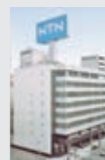
Current head office building
