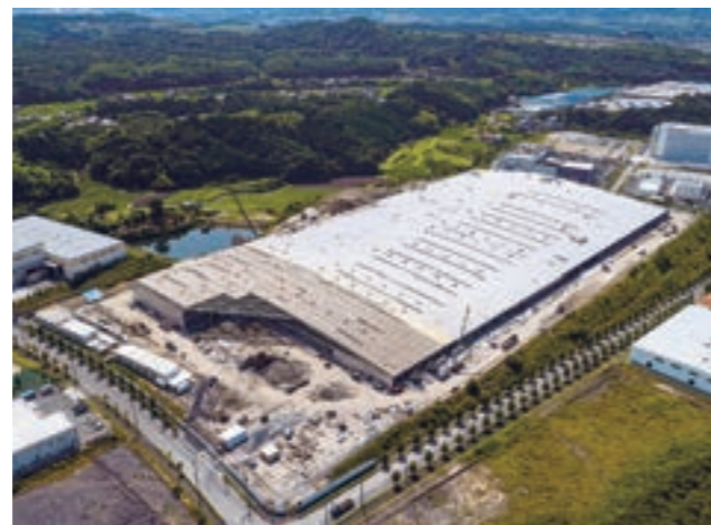
Construction of Wakayama Works in progress (photo taken in July 2019)
