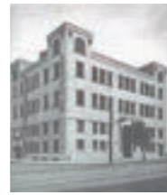
Old head office building
