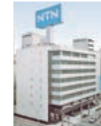
Current head office building
