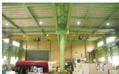
Replacement of mercury lamps with LEDs (NTN SHIKA CORP.)
