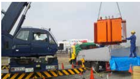
Loading into trucks
