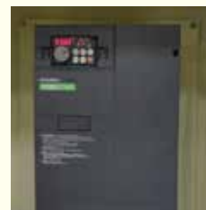
Replacement of pumps with those equipped with inverters (NTN FUKUROI CORP.)
