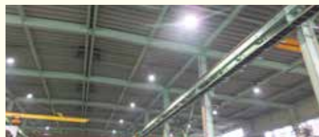
Replacement of mercury lamps with LEDs (NTN HAKUI CORP.)
