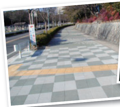
Incinerated ash is recycled into roadbed material like this
