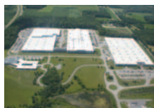
Roofs with heat-reflecting paint
