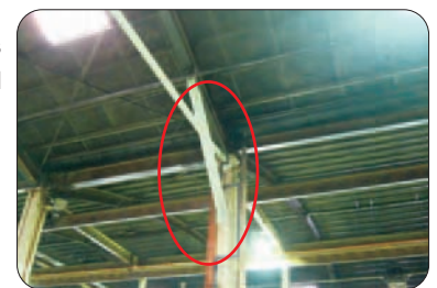
Earthquake resistance improvements underway at Okayama Works
