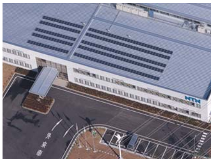
Solar light panels at NTN Fukuroi Corp.
