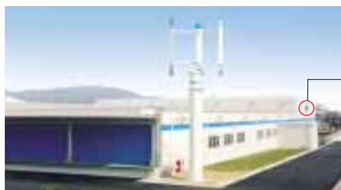
Wind power generator
