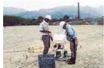
Ground gas investigation
