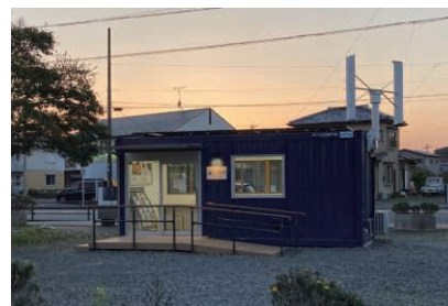
“N 3 N-CUBE” installed as a waiting room at a bus stop in Yoshida Town, Shizuoka Prefecture, Japan
