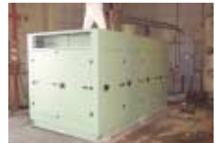
Variable-speed drive scroll compressor
