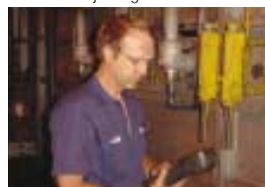
Adjusting the furnace burner
