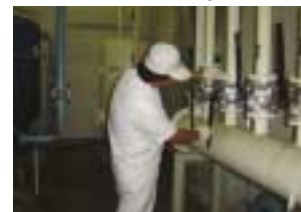
Checking for air leaks
