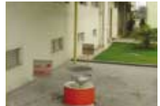
Waste oil storage area
