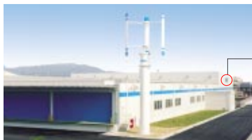
Wind power generator
