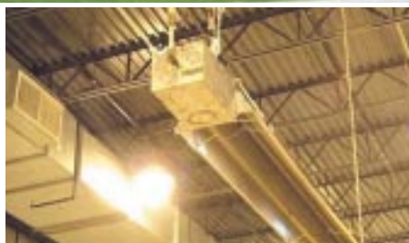
Radiant heaters installed above the work area
