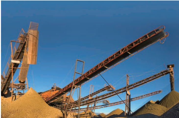
Bulk material conveyors
