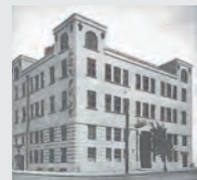
Old head office building
