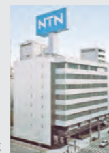
Current head office building
