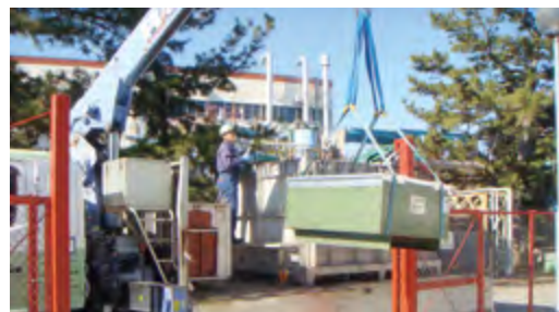
Removal of capacitors containing PCBs
