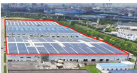
Photovoltaic panels installed on plants
