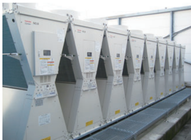
Heat source generation units in the small- and medium-size plant of KUWANA Works
