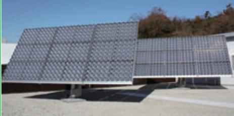
We develop sun-tracking systems and install these so that we can verify and assess their power generation capacity and power consumption.
