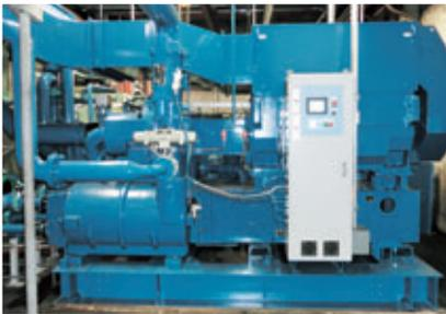
OKAYAMA Works is reducing its CO<sub>2</sub> emissions by upgrading to energy-efficient equipment. The company expects to reduce emissions by 1,560 tons annually through measures including installing high-efficiency air compressors and converting compressor cooling water pumps to inverter types. ⇒p54
