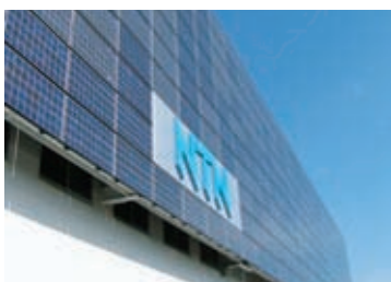
The solar power generation system at Kuwana Works' Extra-Large Bearings Plant 3
