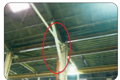
Earthquake resistance improvements underway at Okayama Works
