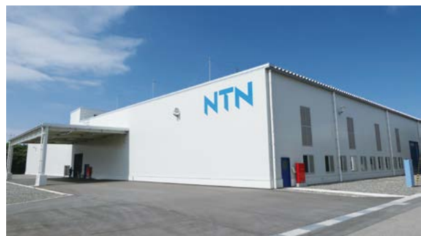
Exterior of heat treatment plant at NTN Noto Corporation
