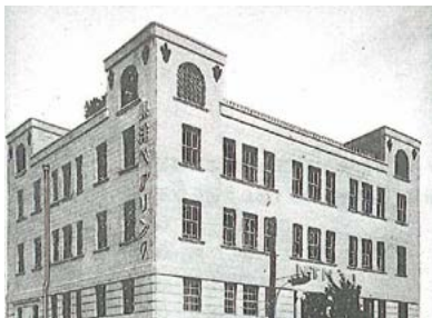
Former head office building
