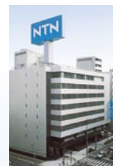
Current head office building
