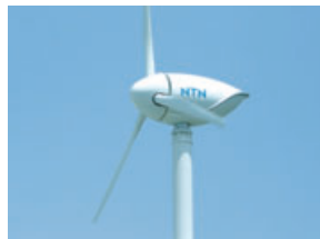
Wind power generator (NTN Houdatsushimizu Corporation)
