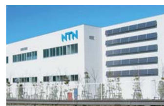
Solar panels at NTN Mie Corp.
