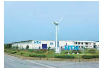
Wind power generator (NTN Houdatsushimizu Corporation)
