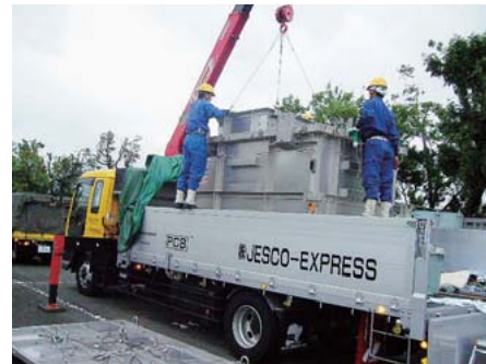
Hauling of PCB devices (former Takarazuka Works)
